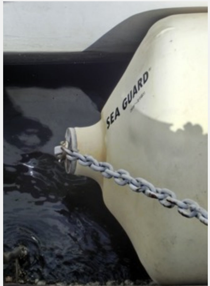
Fender with chains oriented incorrectly. Note damage to the fender ends.
