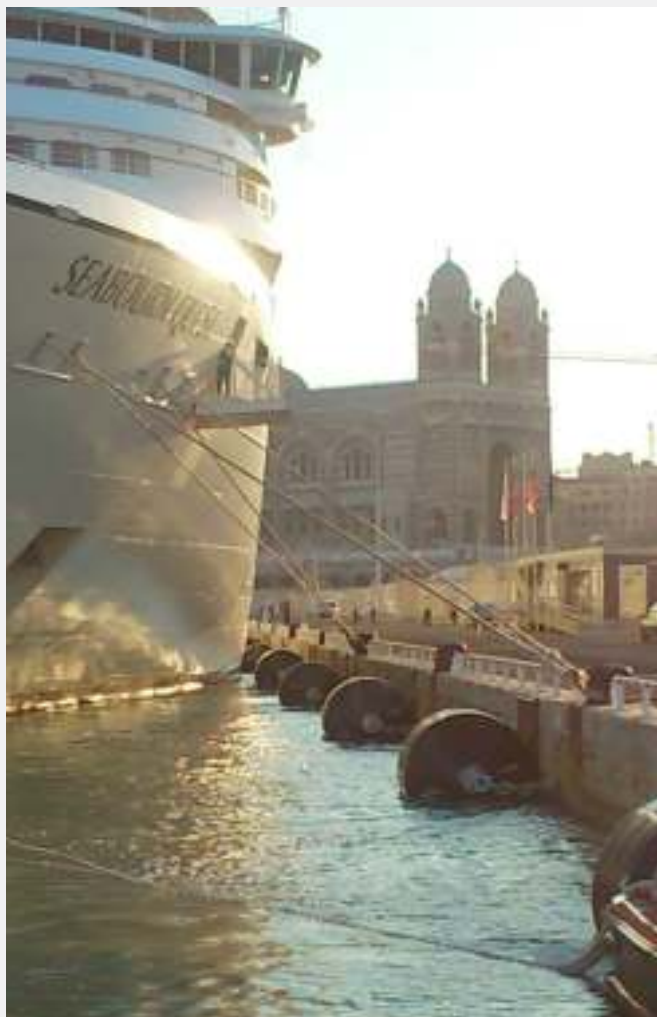
Fender with chains oriented incorrectly. Note damage to the fender ends.
