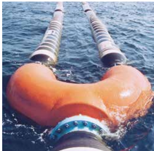
Floating 'Y' Piece on location at Conoco's Tetney oil terminal.
