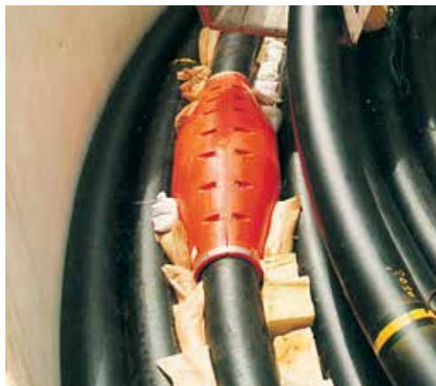
Flange Protector on flexible pipe.
