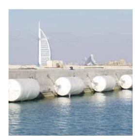
Although rubber fenders remain the preferable solution for some applications, Trelleborg wants to raise awareness of the viable alternative that foam can offer and the applications in which a foam fender might be a more cost effective, low maintenance or quickly installed solution.
