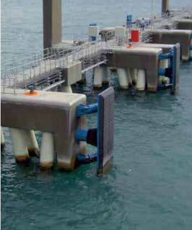
Reverse mounted single cone fender PMF system installed on concrete structure
