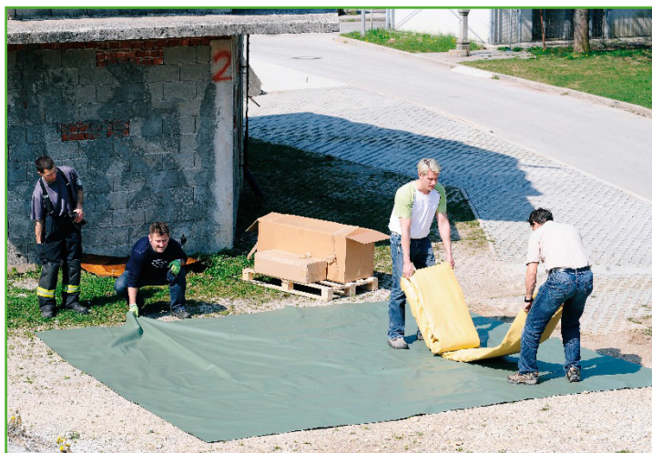
Fig. 5.6: Place the closed rubber tank on the prepared surface
