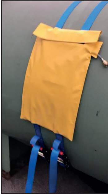
Figure 30: Sealing with using the preprotective bag
