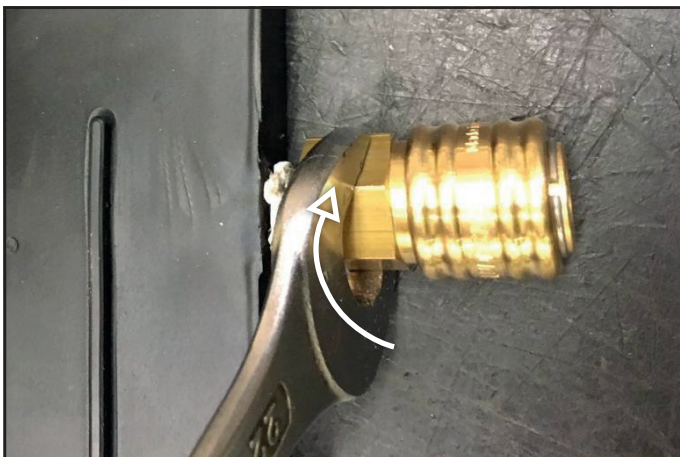
Figure 37: Screwing the new coupling
