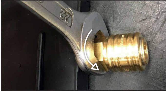
Figure 35: Unscrewing the coupling
