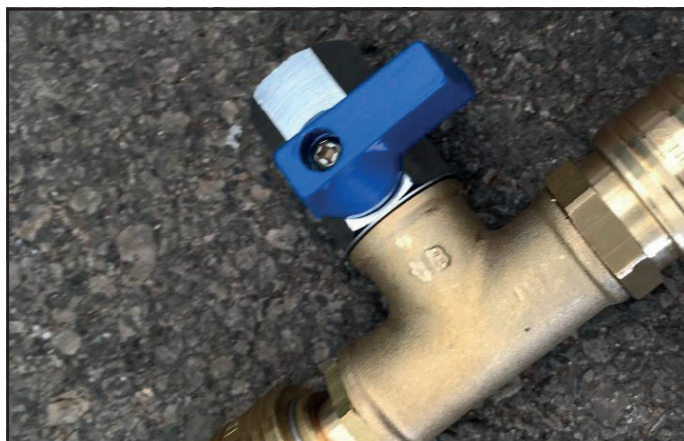
Figure 18: Release valve in closed position
