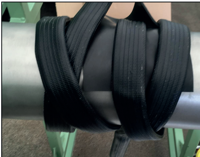
Figure 14: The SAVA sealing tube tied around the damaged object
