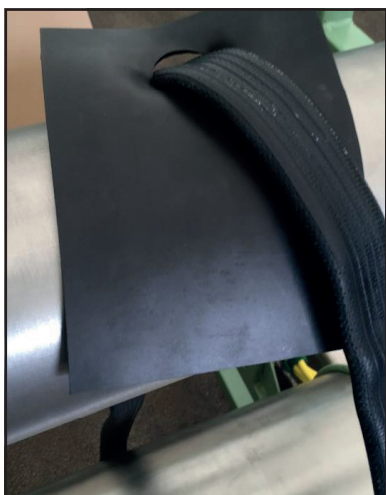
Figure 12: The sealing plate positioned on the damaged area
